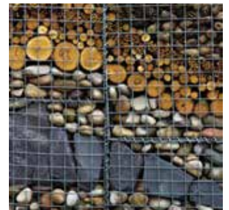
Gabion baskets - mixed fill
